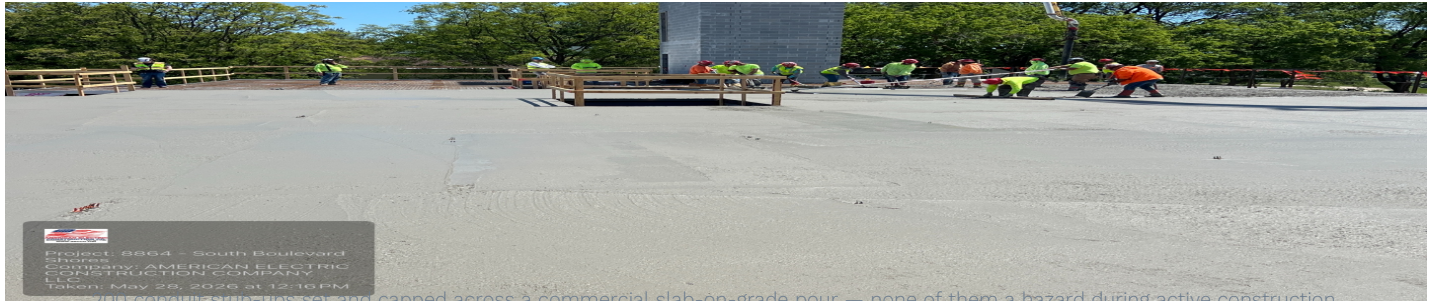
200 conduit stub-ups set and capped across a commercial slab on grade pour — none of them a hazard during active construction.
